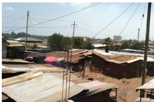
The semi-permanent housing structures
