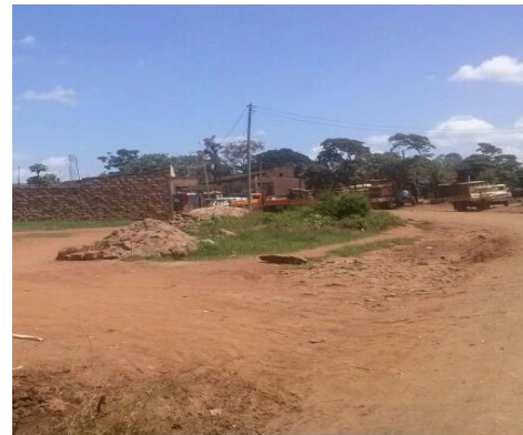
Exposed Surface- Source of Air Pollution
