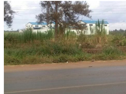
Building Constructed in a Wetland
