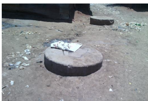
The sewer line - Manholes
